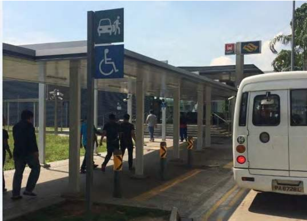
PasirPanjang MRT Taxi Stand (In-front of Pasir Panjang Food Centre)
